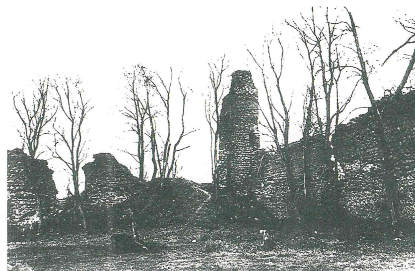
Fig. 2. The north-east corner of the Medininkai castle before conservation (1958), photo: M. Sakalauskas
