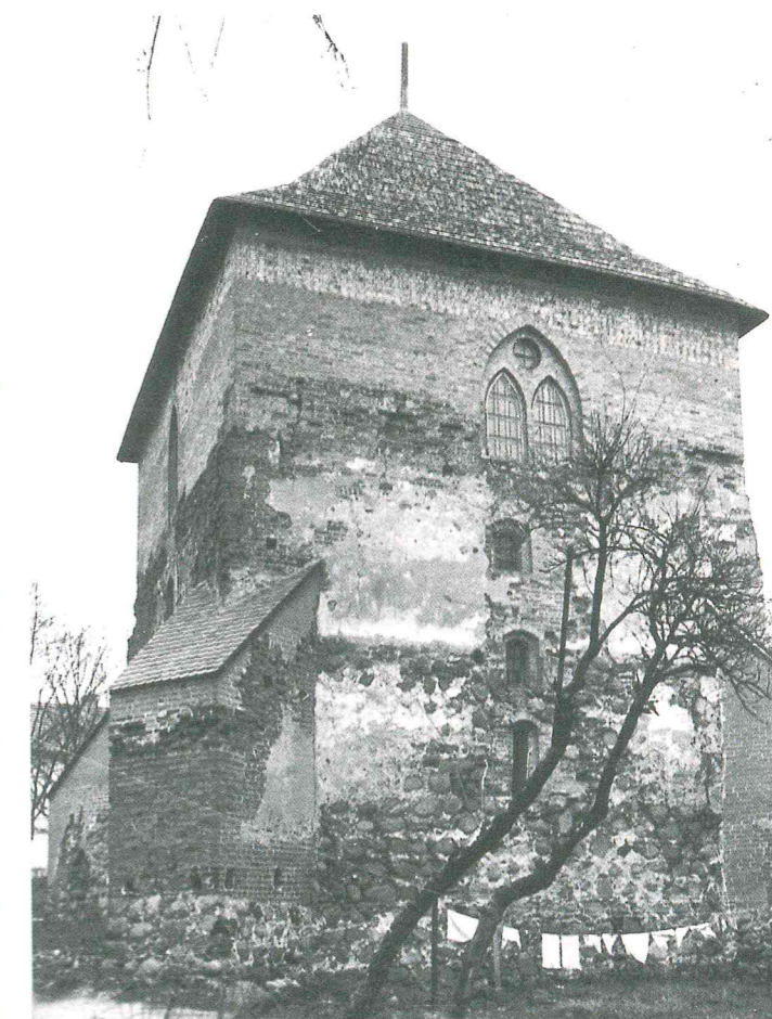
Fig. 5. Trakai peninsular castle, southern tower (1996)
